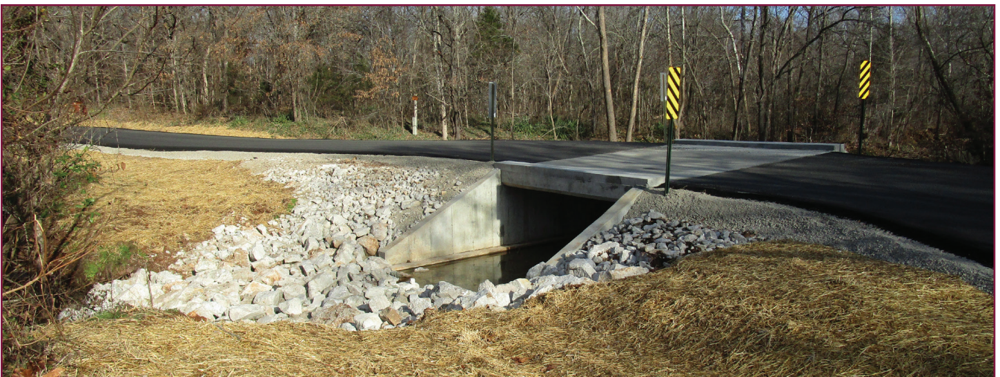
MRPC continued administering a DRA grant to replace the bridge over Mill Creek in Washington County. The bridge was completed in December 2024.
