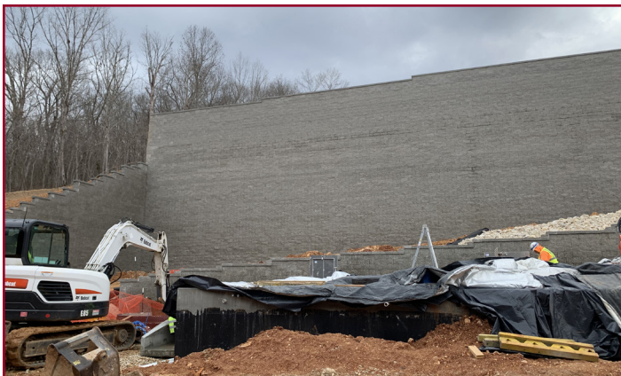
MRPC's grant administration staff continued work on administering a Community Development Block Grant for $3.5 million to St. Robert for the construction of a wastewater treatment facility. Construction is currently in the fourth phase.
