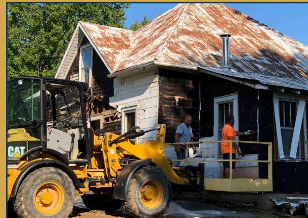
Left: Crews with Central Missouri Excavating Company began prepping a house in Belle for demolition by removing siding. Belle received a Community Development Block Grant to demolish seven vacant and dilapidated residential structures around the city.
