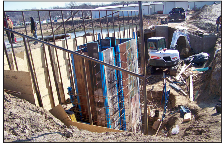
Right: Crews from Mid-State Pipeline Maintenance of Belle work on digging and setting forms for the new UV disinfectant treatment system near the lagoons at the Chamois waste water treatment facility on Jan. 30, 2018. The project cost approximately $1.9 million.
