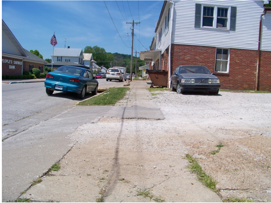
Fair Condition: West Fifth Street, north side looking west
