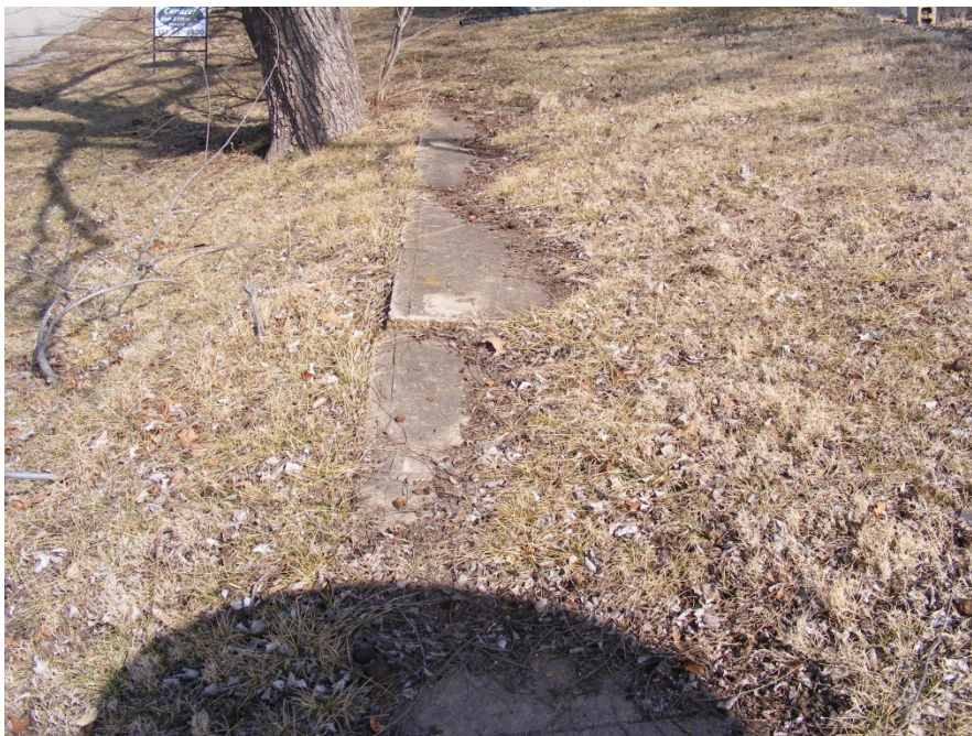
Poor Condition: N.W. corner of Taylor and East Missouri, looking north
