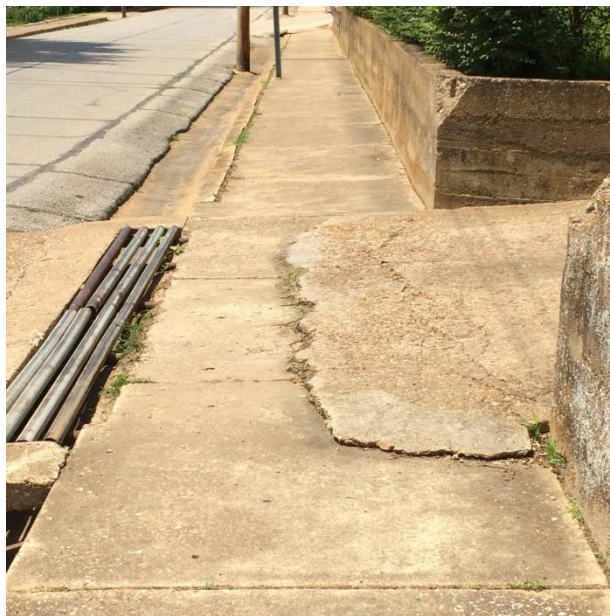
Poor Condition: East side of East Main close to downtown.
