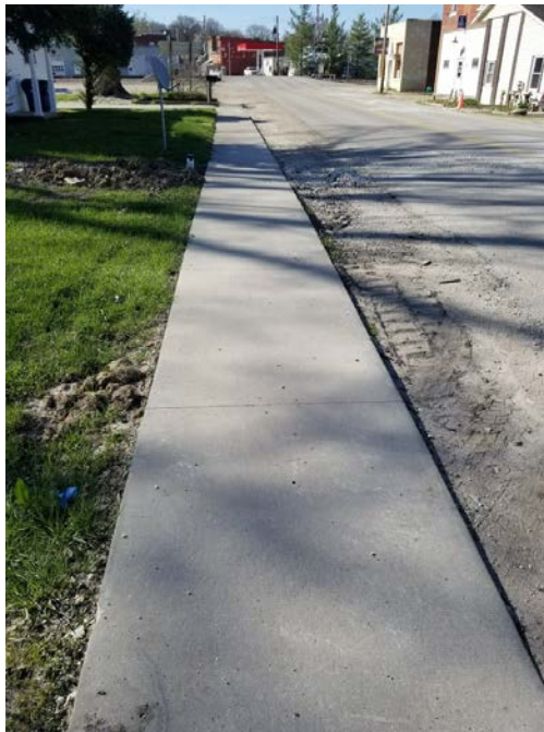
Good Condition: Main Street, east side looking south towards railroad tracks.
