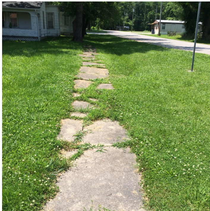
Poor Condition: Located at 2 nd and Bertha streets.
