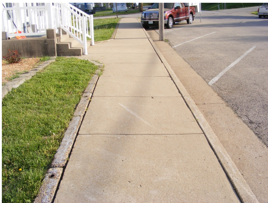
Good Condition: N. Main Street, west side looking north toward 6 th Street
