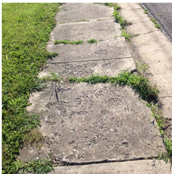
Poor Condition: South side of 2 nd Street from Hwy. 532 to Pine Street.
