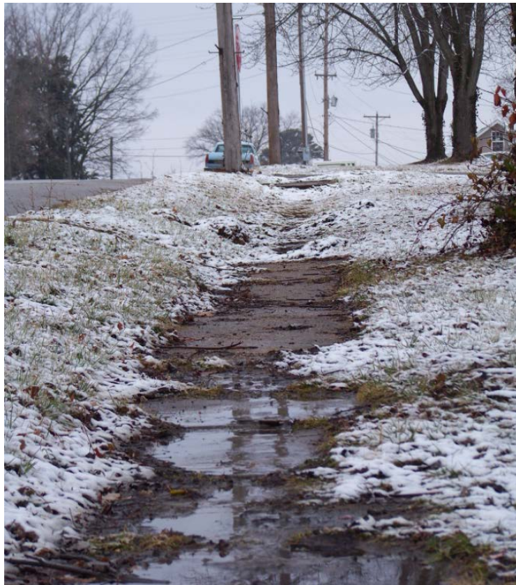
Poor Condition: Washington Blvd, north side looking west
