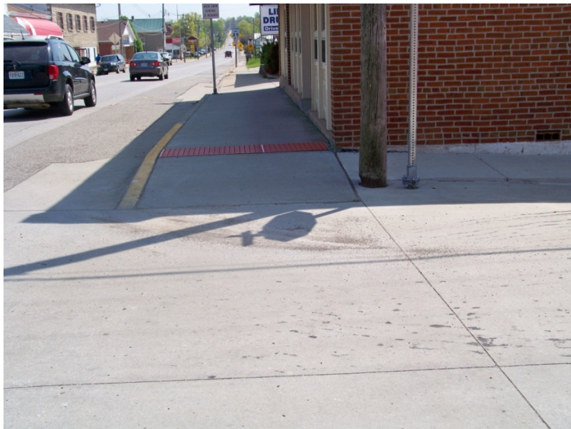
Good Condition: Corner of U.S. Hwy 50 (Main) and Third Street, south side looking east
