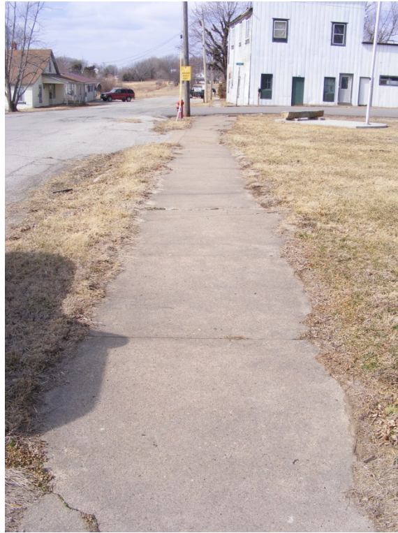
Fair Condition: North side of W. Colorado Ave., looking west to Frost Street
