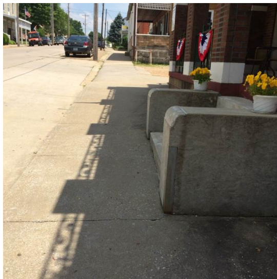
Good Condition: West side of East Main between Maries and Mill streets.
