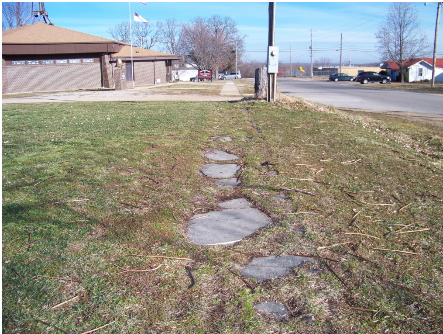
Poor Condition: S. Walnut Street, west side looking north
