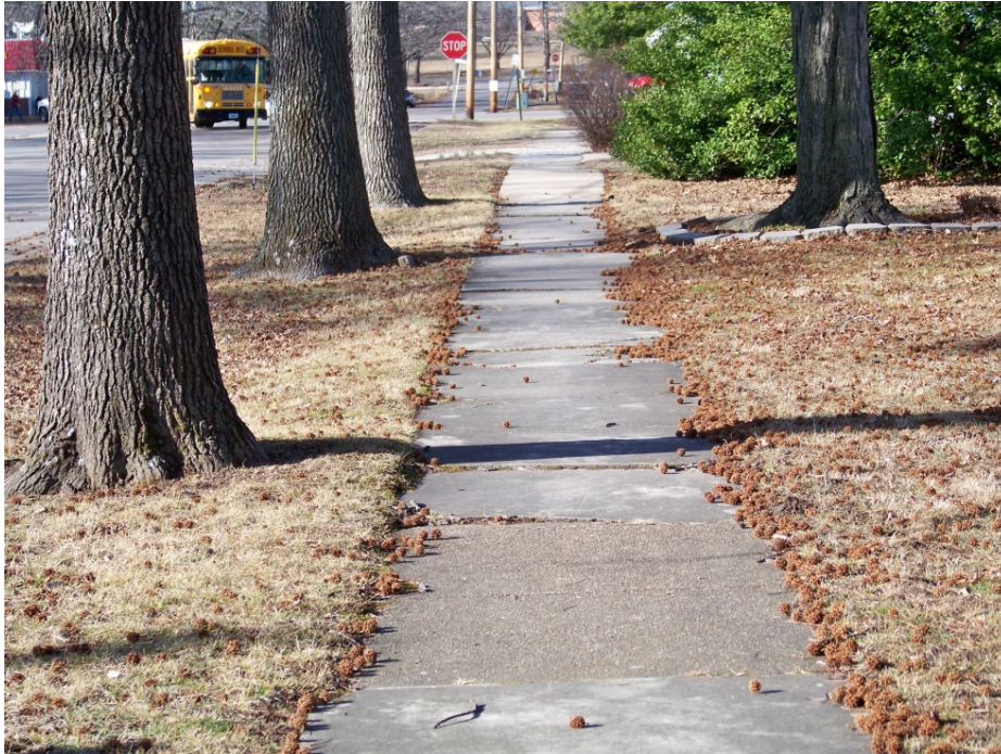
This sidewalk, in fair condition, is located on Seymour Street.
