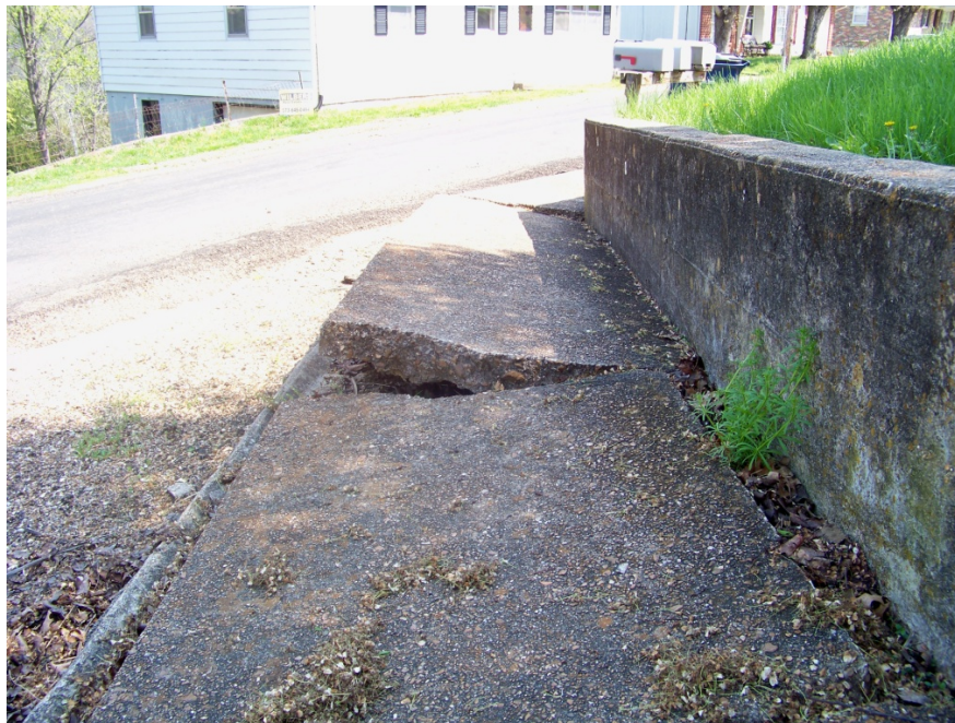
Poor Condition: Corner of Benton Street and Fifth Street, south side
