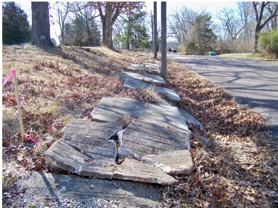
Poor Condition: Taylor Street, east side looking south
