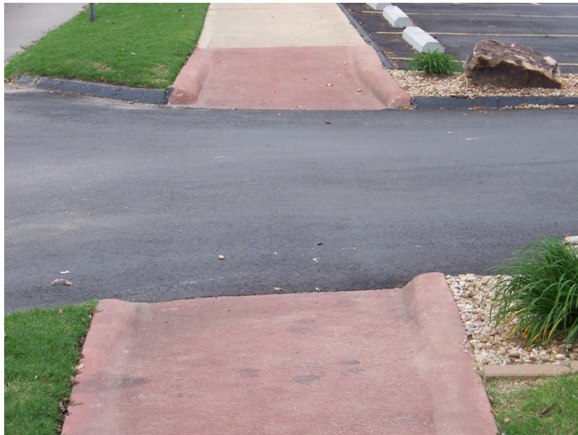
Good Condition: Main Street, south side looking east toward S. 4 th Street
