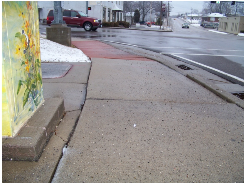
Good Condition: Intersection of North Franklin St and West Washington Blvd
