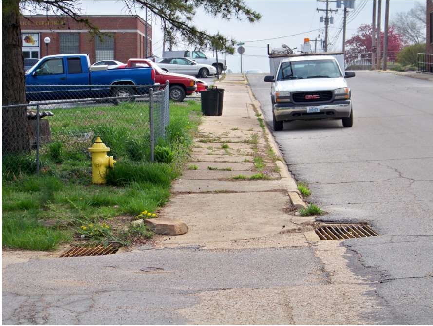
Fair Condition: Intersection of N. Henderson and 5 th Street, north side looking west
