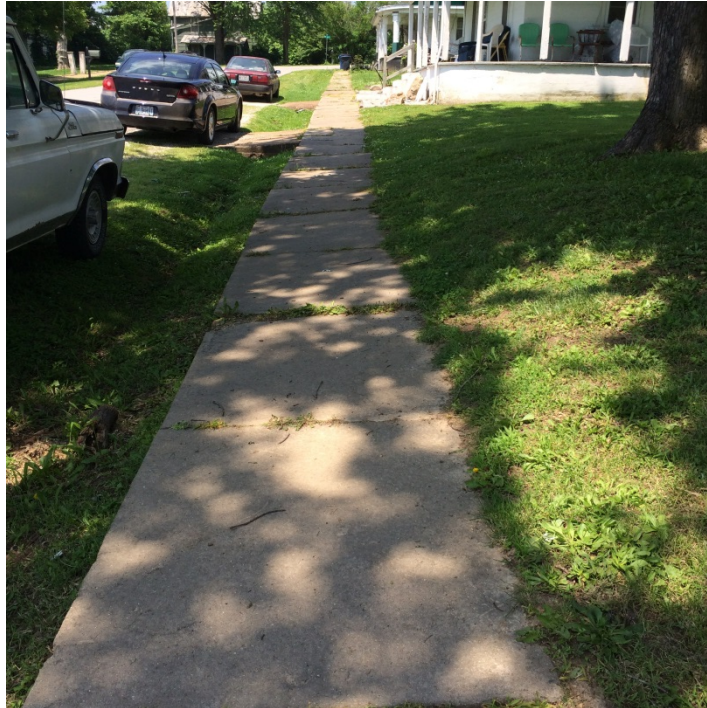
Fair Condition: West end of 5 th Street
