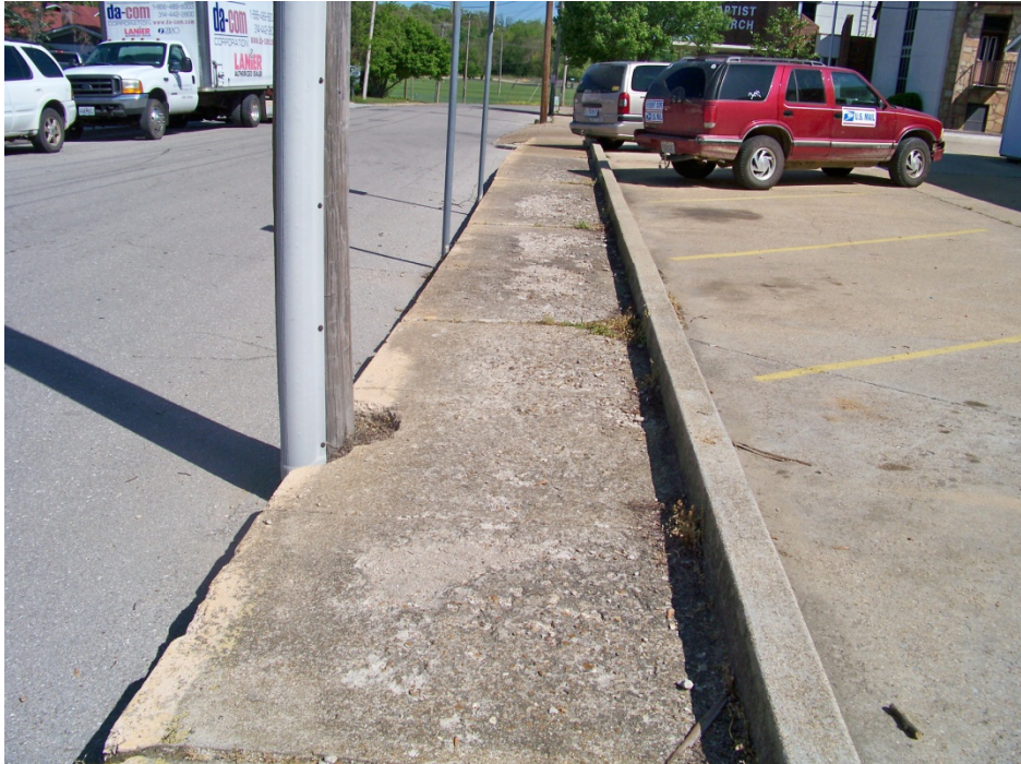
Fair Condition: North Benton Street, east side looking north
