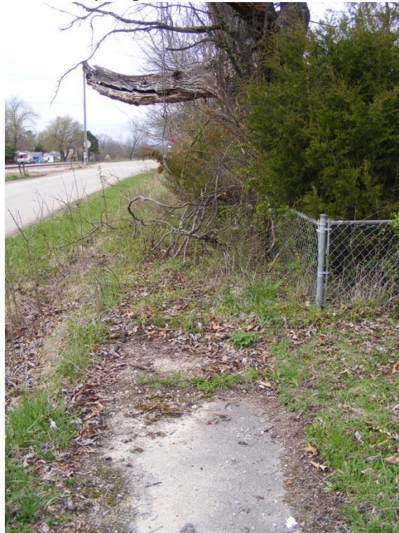
Poor Condition: North side of E. Springfield Avenue looking southwest.
