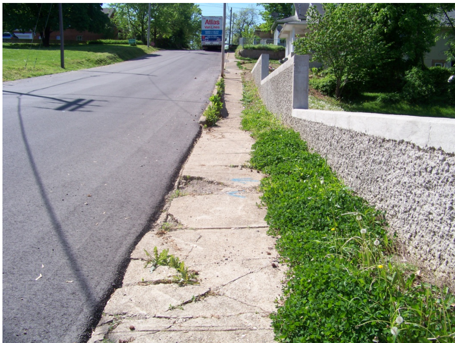
Poor Condition: South Benton Street, west side looking south
