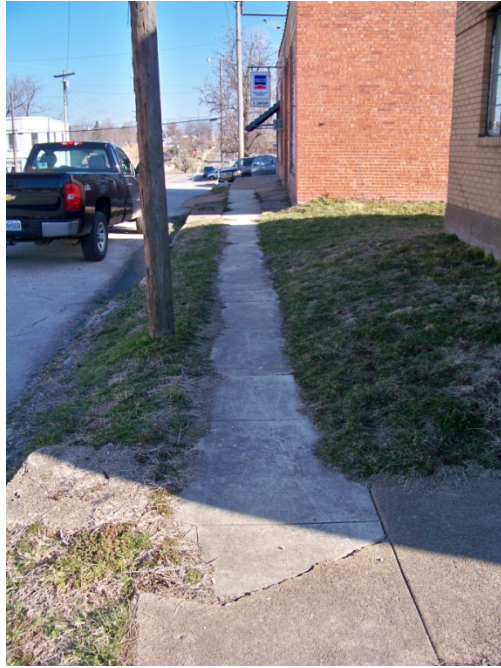
Fair Condition: North Commercial Street, east side looking north
