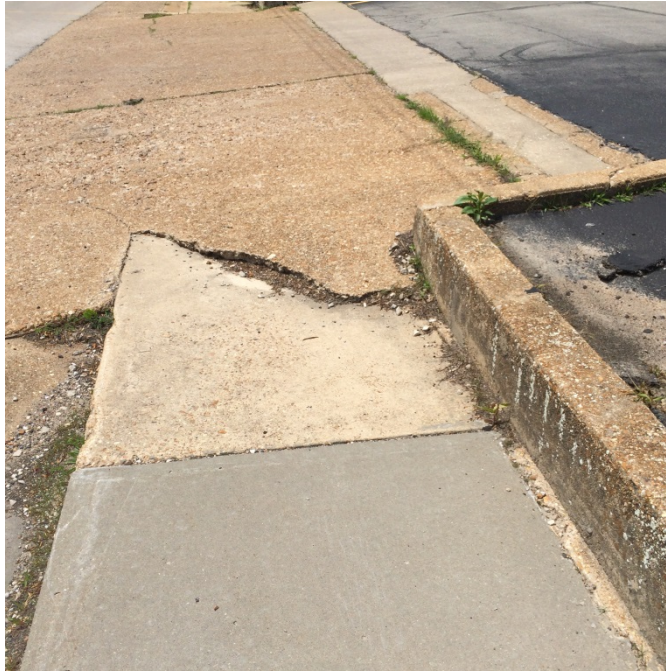
Fair Condition: East side of East Main close to downtown.
