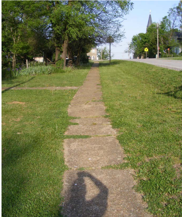
Fair Condition: 5 th Street, south side looking west
