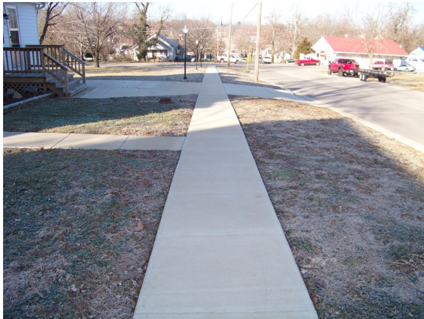
Good Condition: E. 3 rd Street, south side looking west
