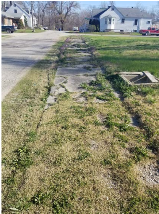
Poor Condition: Main Street, north of Missouri Avenue looking north.
