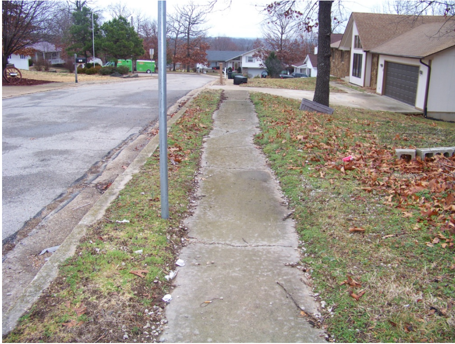
Fair Condition: Woodland Lane, south side looking east
