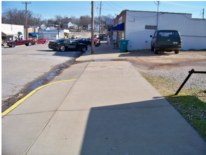
Good Condition: E. Pine Street, south side looking east toward Walnut Street
