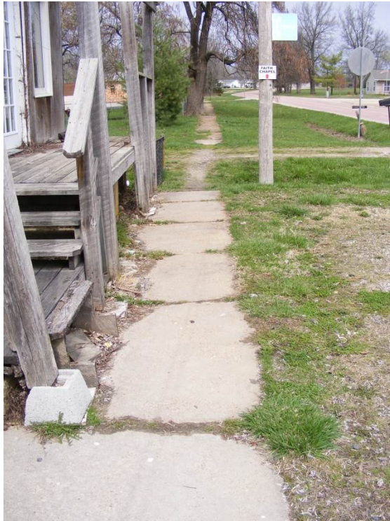
Fair Condition: Intersection of Springfield Avenue and Second Street looking northwest.
