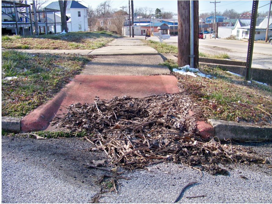
Fair Condition: Intersection E. Pine Street and Olive Street, southeast corner
