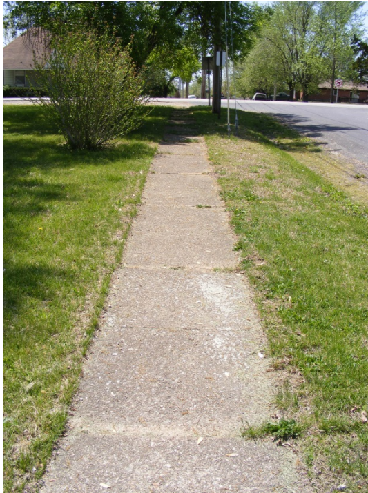
Fair Condition: Cedar Street, east side looking south toward Highway 50.
