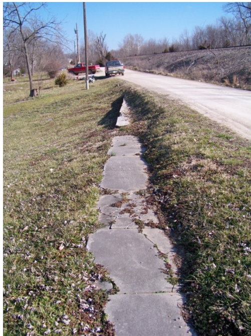
Poor Condition: Eastside Street, west side looking north
