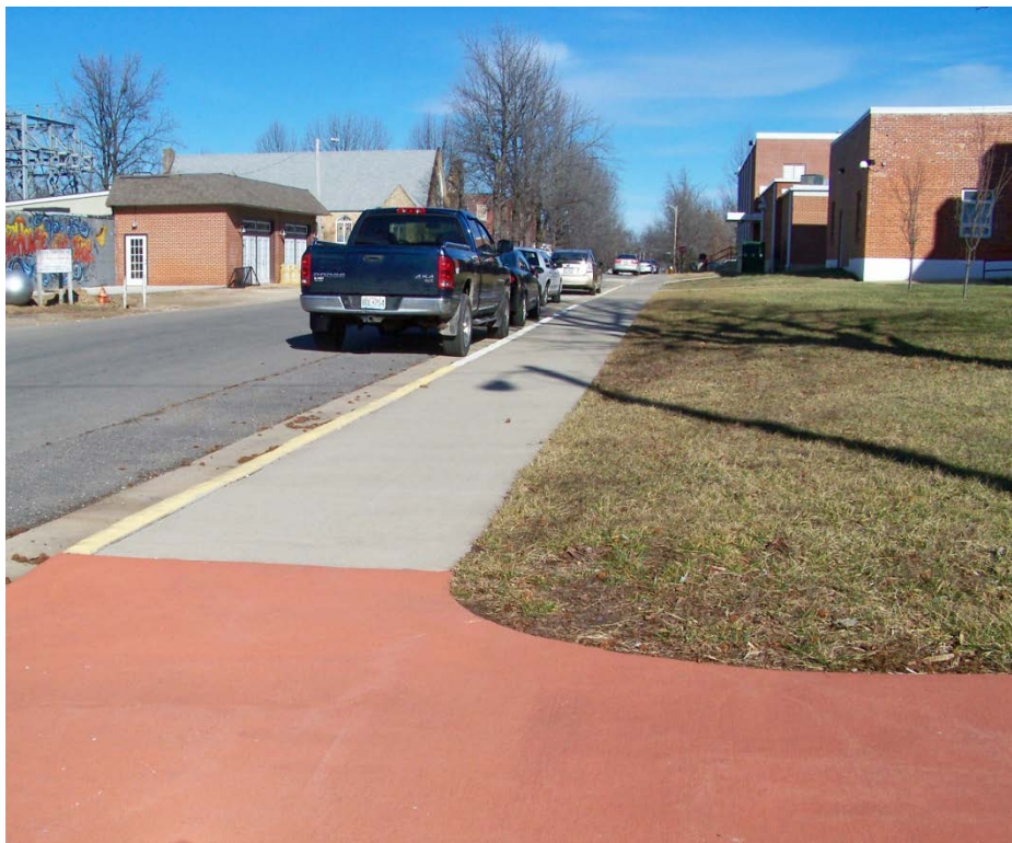
This sidewalk, located on the north side of Washington Street, is in good condition.
