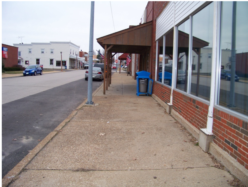
Good Condition: S. 1 st Street, west side looking south toward E. Washington Avenue
