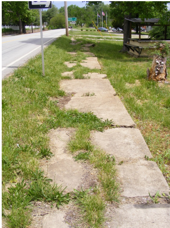
Poor Condition: Main Avenue (Hwy 21), west side looking north.
