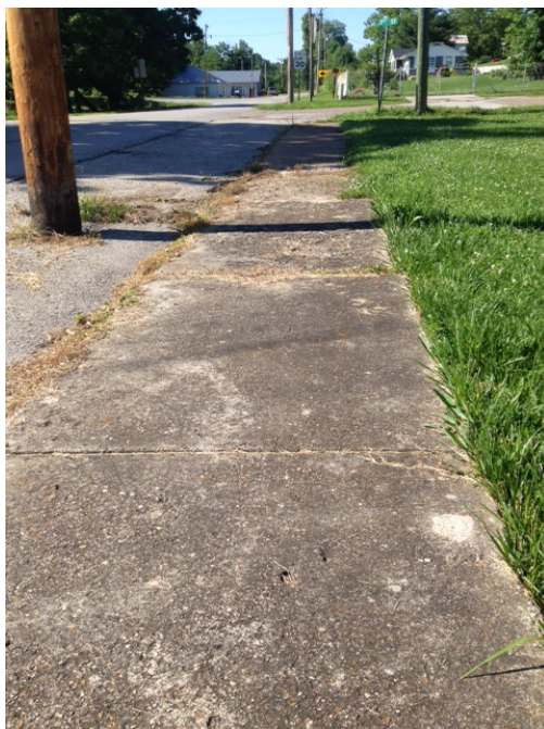
Fair Condition: East side of Hwy. 532 from 2 nd to 3 rd Streets.
