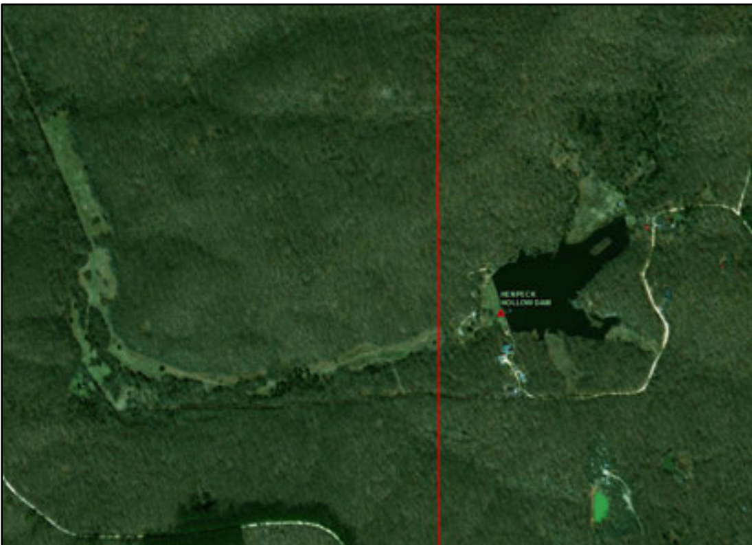
Figure 3.11. Henpeck Hollow Dam
