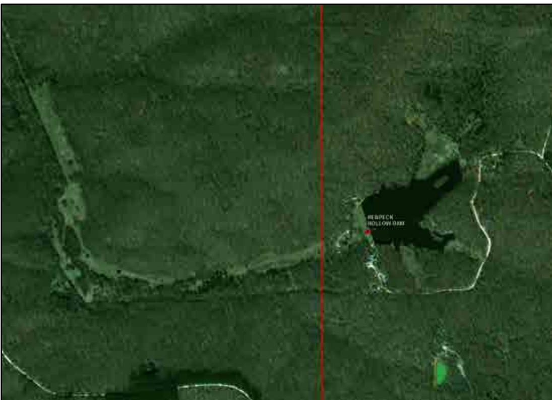
Figure 3.11. Henpeck Hollow Dam
