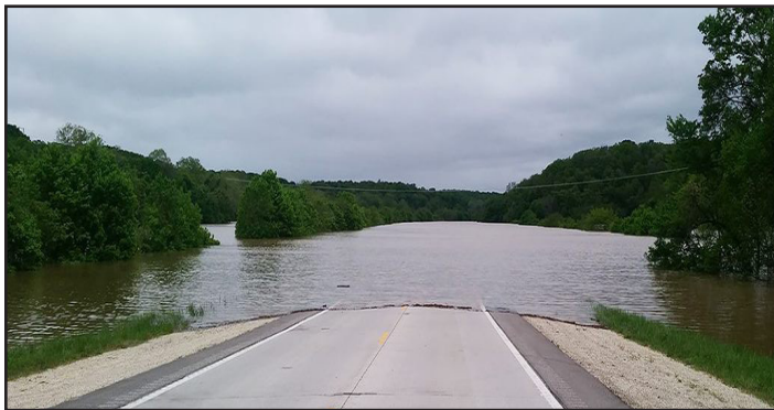
Flooding in April and May of 2017 blocked off many of the major roadways in the Meramec Region. Above water covers Hwy 63 near Vienna. Many of the roadways remained closed for days.
