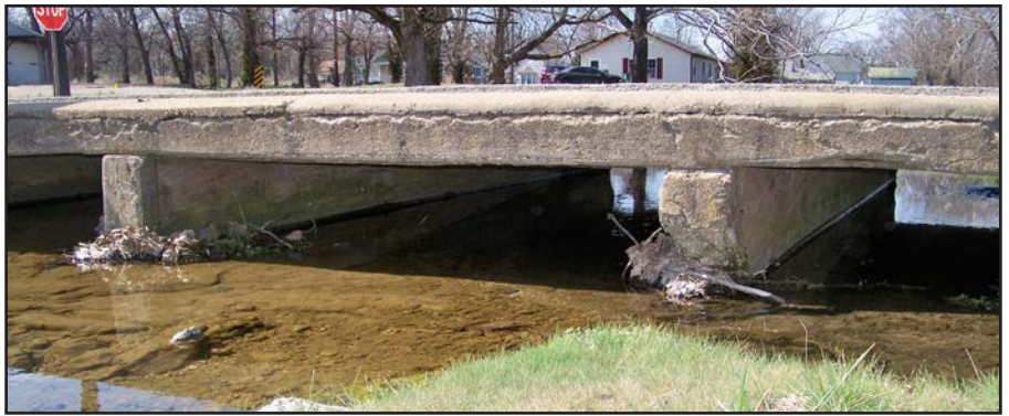
The City of Potosi was awarded $389,723 to replace the Mill Street Bridge over Breton Creek. After 50 years of use, the supports under the bridge have begun to crumble.
