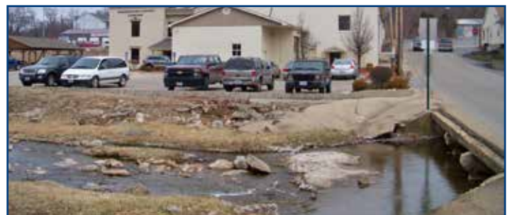
MRPC staff worked closely with Potosi officials to submit a CDBG grant to help fund a bridge project on Mill Street.
