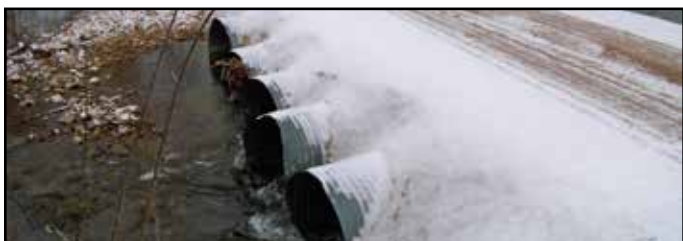
MRPC staff worked closely with Washington County officials to submit a CDBG grant to replace a low water crossing in Washington County.
