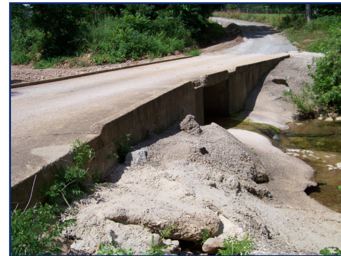
BRIDGE 11 Robinson Road
