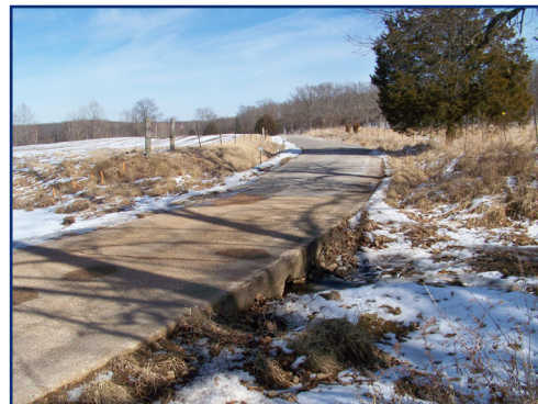
BRIDGE 13 Springfield Road
