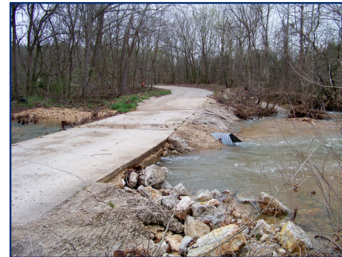
BRIDGE 5 Goose Creek Road 303
