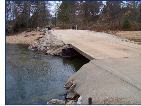
BRIDGE 4 Sellers Road
