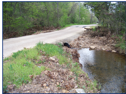
BRIDGE 8 Simpson Road 334
