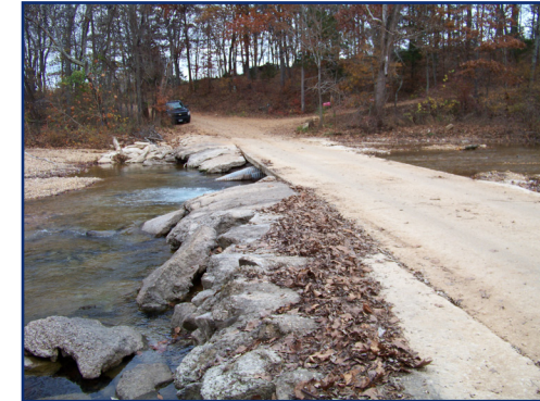
BRIDGE 5 Wilhite Road
