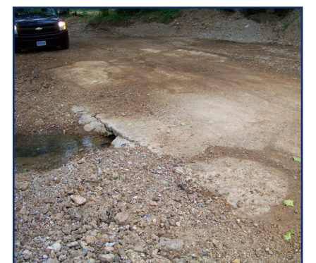
BRIDGE 19 Keith Cemetery Road
