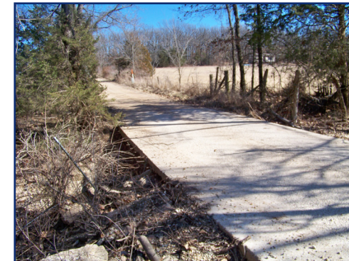
BRIDGE 16 Ware Road
