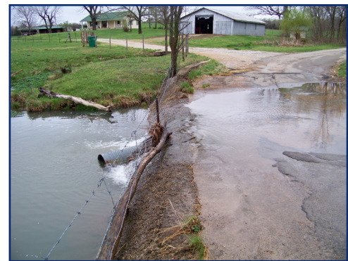
BRIDGE 7 Lick Skillet Road 320
