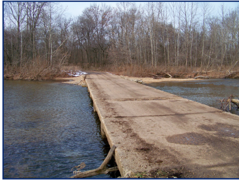
BRIDGE 1 Westover Road
