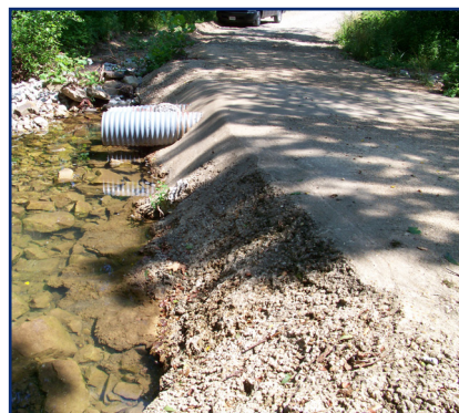
BRIDGE 16 Carr Road 535
