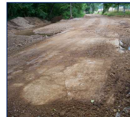
BRIDGE 18 Cubb Creek Road 650
