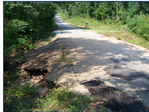
BRIDGE 9 Duncan Road 343
