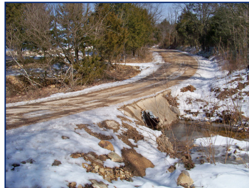
BRIDGE 14 Hinch Road
