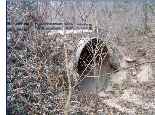
BRIDGE 11 Rock Road
