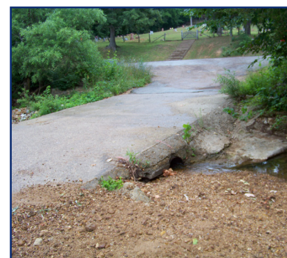
BRIDGE 17 Cubb Creek Road 650
