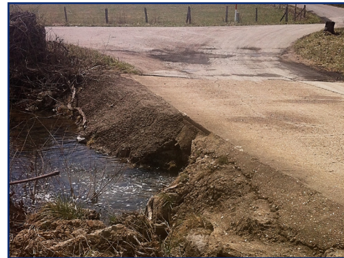
BRIDGE 10 Pelican Ridge Road 304
