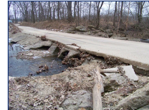
BRIDGE 17 4 Mile Road
