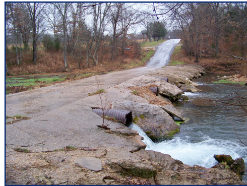
BRIDGE 8 Westover Road
