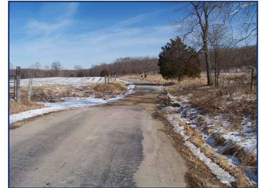
BRIDGE 12 Springfield Road
