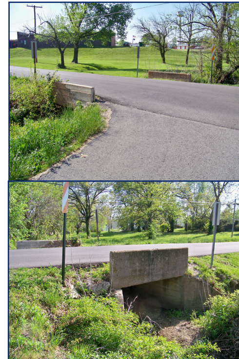
BRIDGE 11 Fifth Street—Belle
