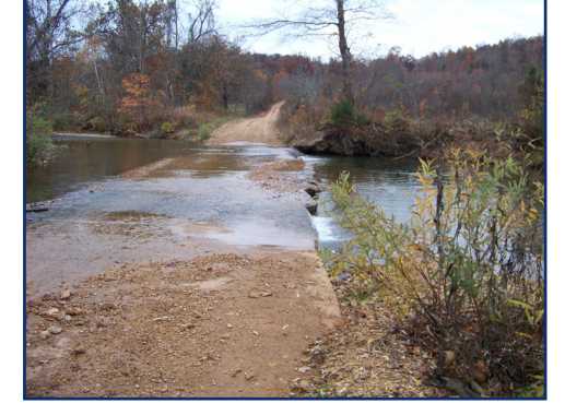
BRIDGE 6 Wilhite Road
