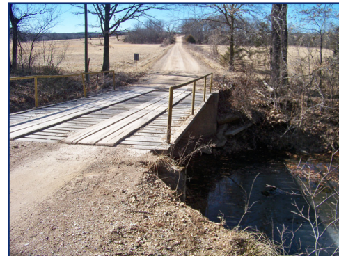
BRIDGE 15 Smith Road
