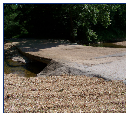
BRIDGE 15 King Road 622
