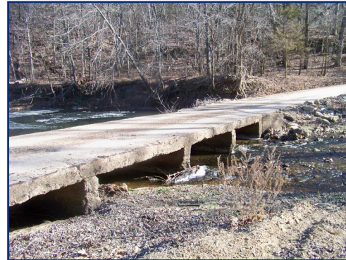
BRIDGE 9 High Point Road
