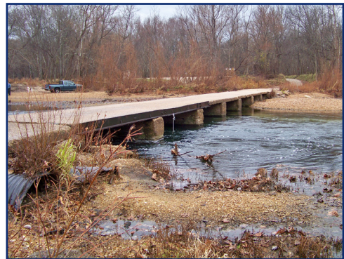
BRIDGE 7 Thurman Lake Road
