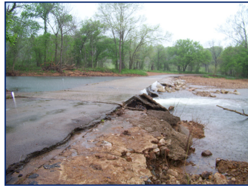
BRIDGE 1 Tiff Road 408
