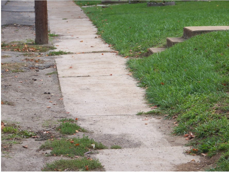
Fair Condition: E. Jefferson Street between S. Water Street and Mill Street, looking southeast
