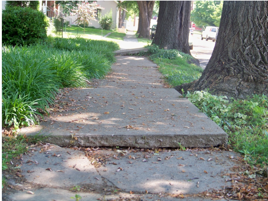
Poor Condition: West Third Street, north side looking east
