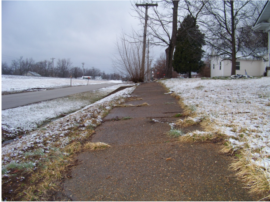
Fair Condition: West Main Ave, north side looking west
