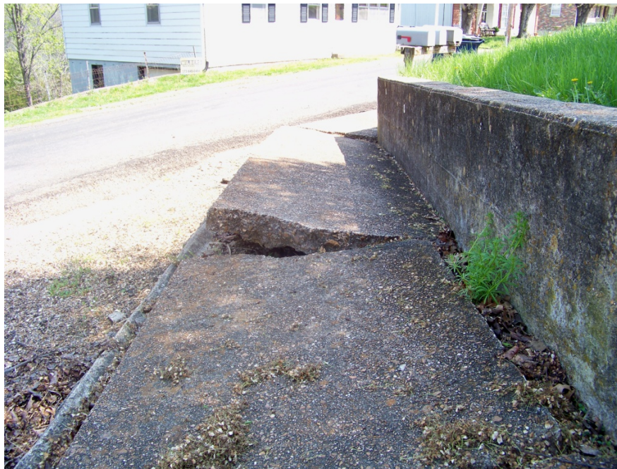
Poor Condition: Corner of Benton Street and Fifth Street, south side
