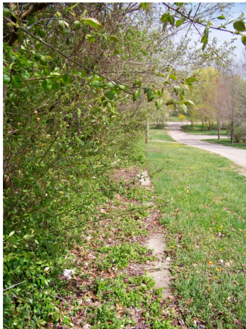
Poor Condition: N. Main Street, east side looking north (adjacent to historical marker)
