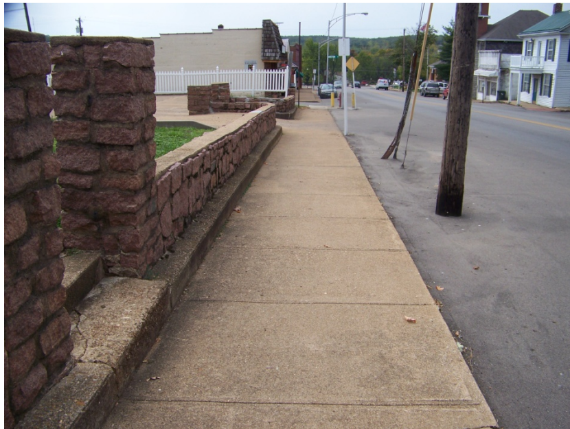
Good Condition: N. Missouri Street, between Brenton Street and Hickory Street looking west
