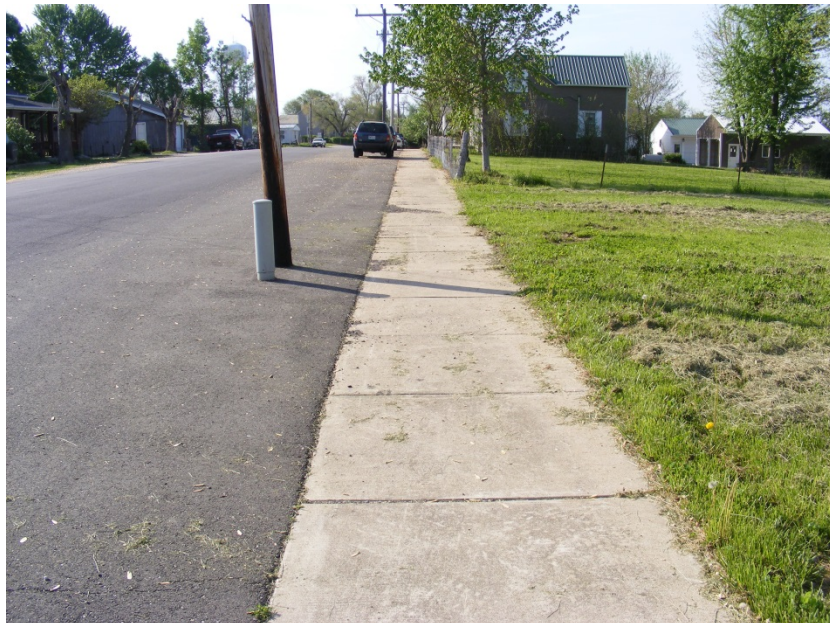
Good Condition: Holy Family Road, west side looking south.
