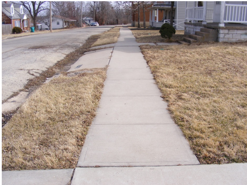
Good Condition: E. Kansas City Street, south side looking east from Main Street
