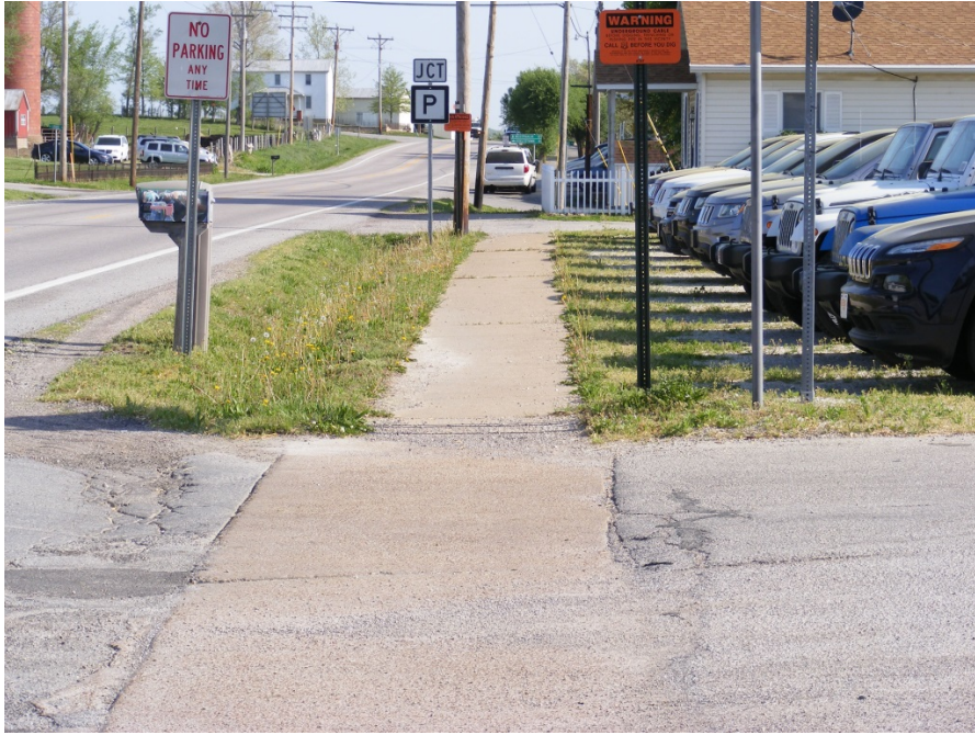
Fair Condition: Locust Street (Highway 63), west side looking north.
