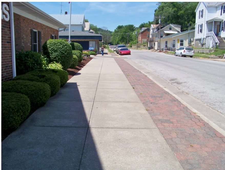
Good Condition: West Fifth Street, south side looking west
