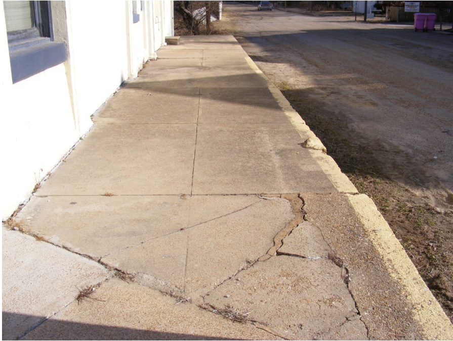
Fair Condition: N.W. corner of Front Street and Water Street, looking north
