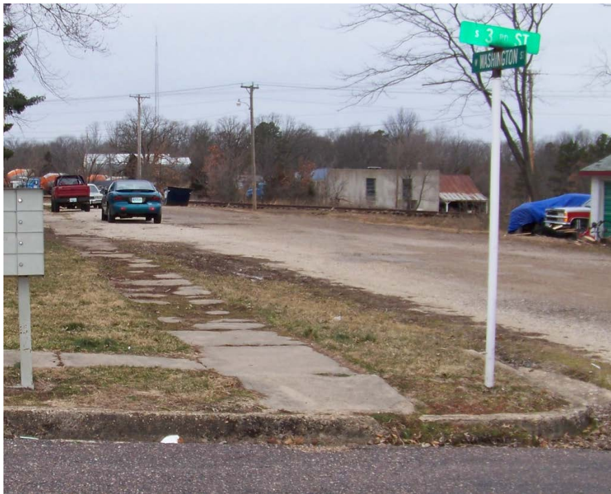
Poor Condition: W. Washington Avenue west of S. 3 rd Street, south side looking west
