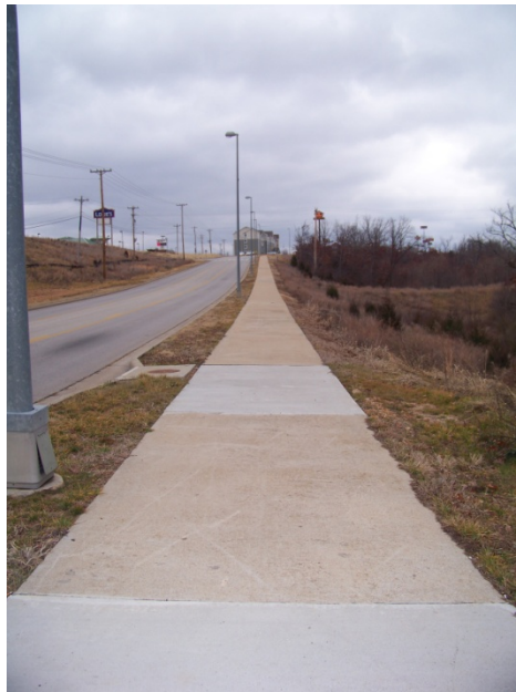
Good Condition: St. Robert Boulevard, south side looking east
