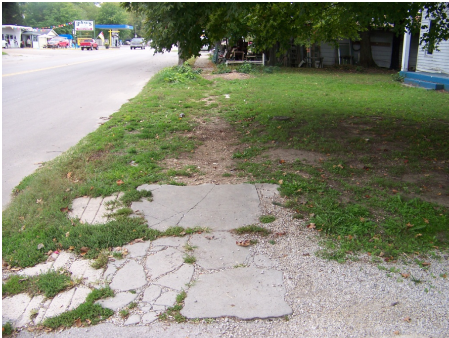
Poor Condition: Main Street, north side looking west toward S. Spring Street
