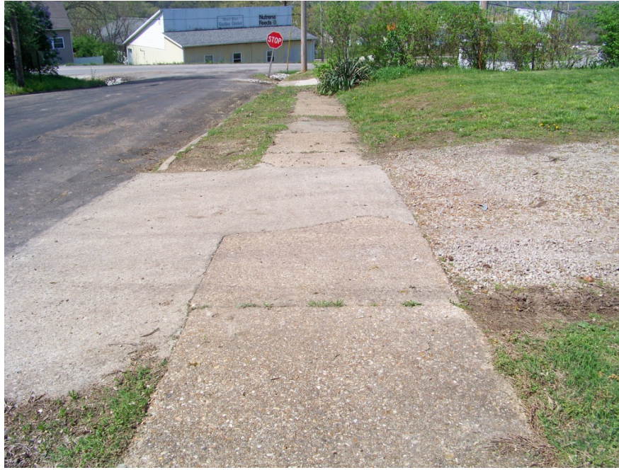
Fair Condition: Benton Street, north side looking west
