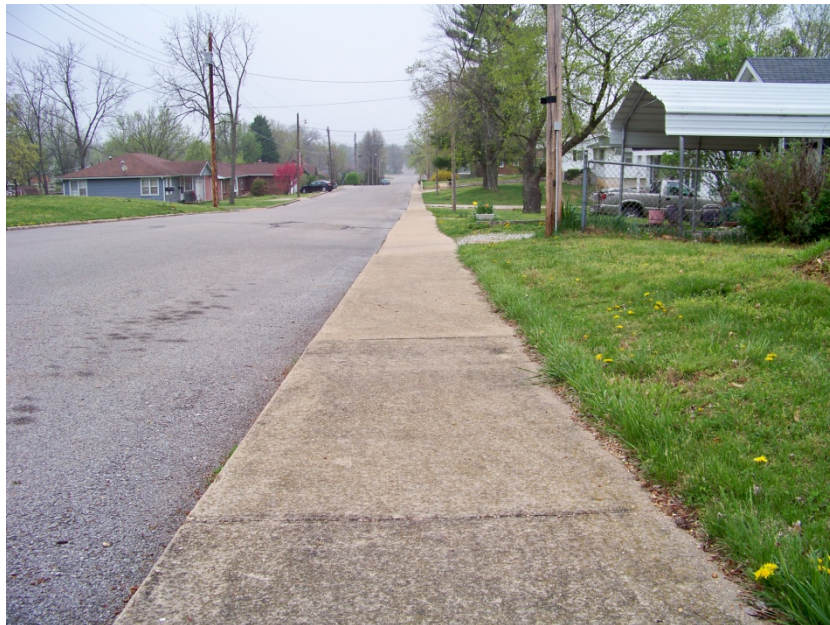
Good Condition: South end of Jackson Street, east side looking north
