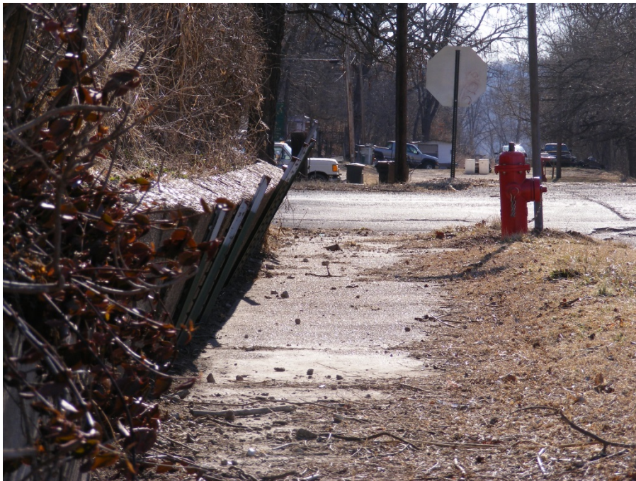
Poor Condition: N.W. corner of Front Street and Hollow Street, looking east
