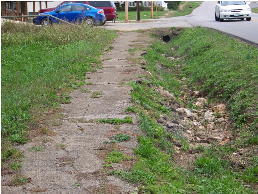
Poor Condition: N. Missouri Street between Rosemary Ave and Cordia Ave, looking northeast
