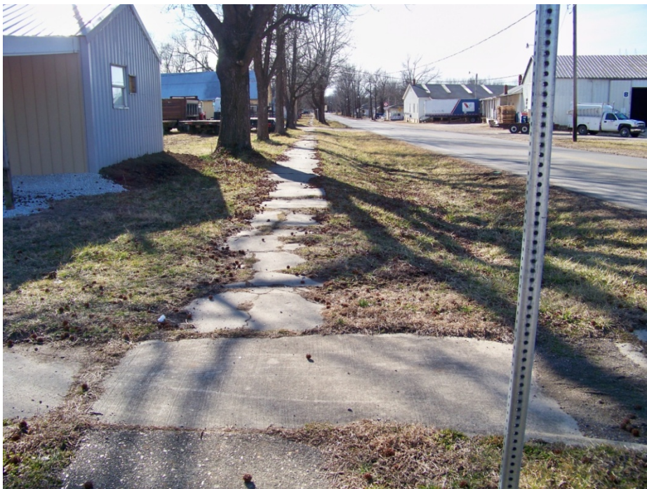
A large portion of the sidewalks in St. James are in poor condition, such as these along W. Washington Street.
