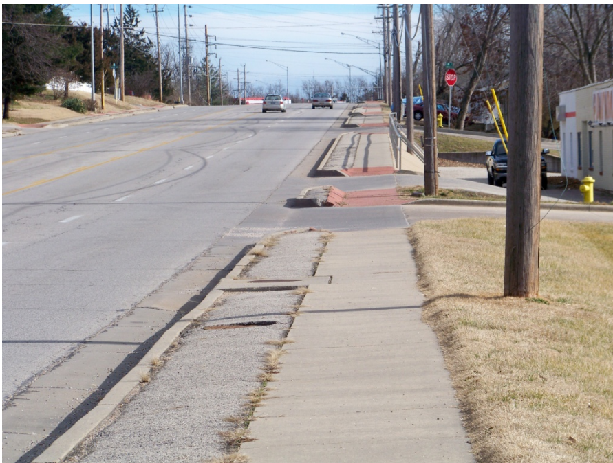
This sidewalk, located on the south side of Hwy. 72, is in good condition.
