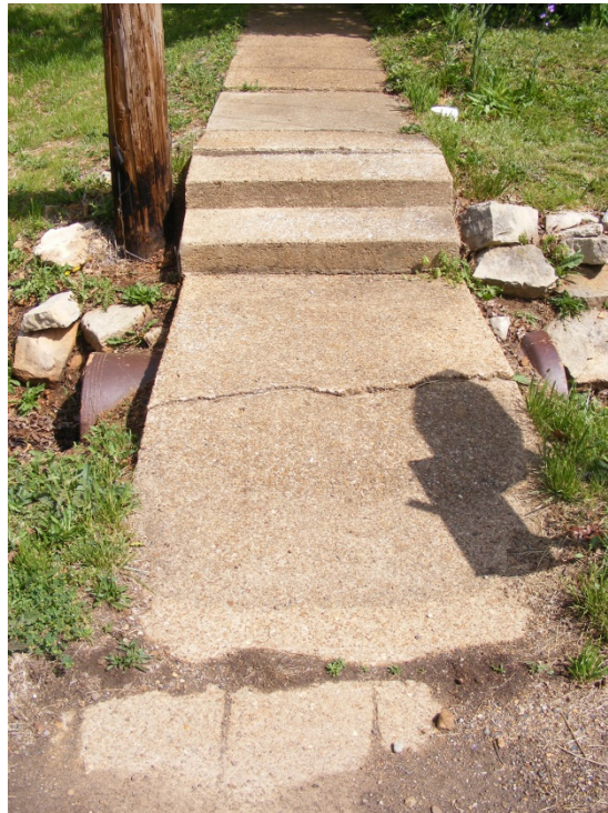
Poor Condition: Intersection of Ash Street and Linden Street, northeast corner looking north.
