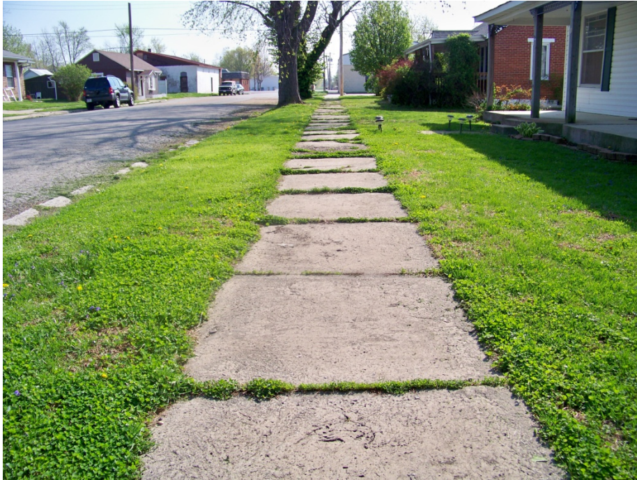
Fair Condition: Second Street, south side looking east
