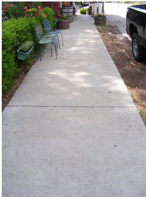
Good Condition: Main Avenue (Hwy 21), east side looking south toward Alexander Street.
