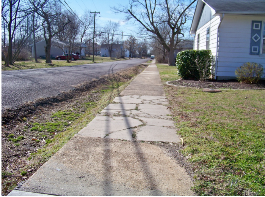
Fair Condition: Taylor Street, west side looking south
