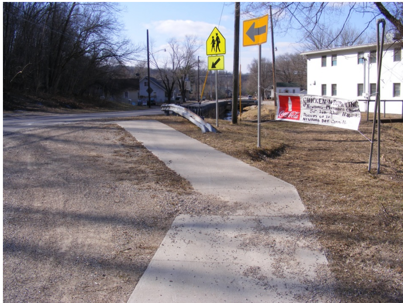
Good Condition: School crossing west side of Main Street (Highway T) near the intersection of Wolf Pride Drive
