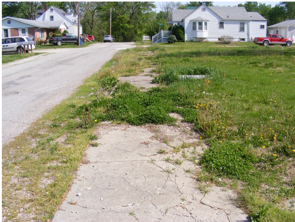
Poor Condition: Main Street, north of Missouri Avenue looking north.
