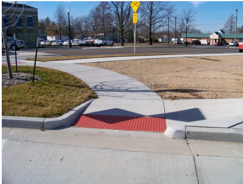
Good Condition: Roundabout at intersection of Taylor and Washington
