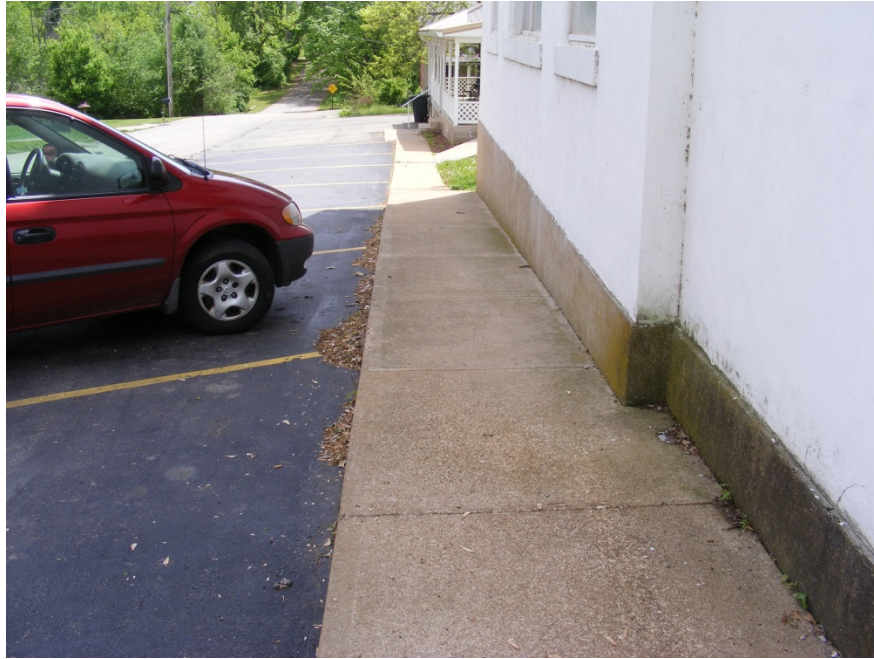
Fair Condition: Alexander Street, south side looking east toward College Street.
