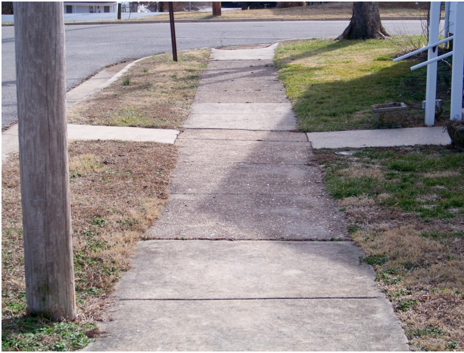
This sidewalk, in fair condition, is located on Cedar Street.
