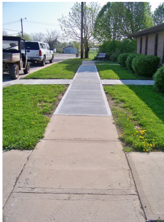
Good Condition: Third Street, south side looking east
