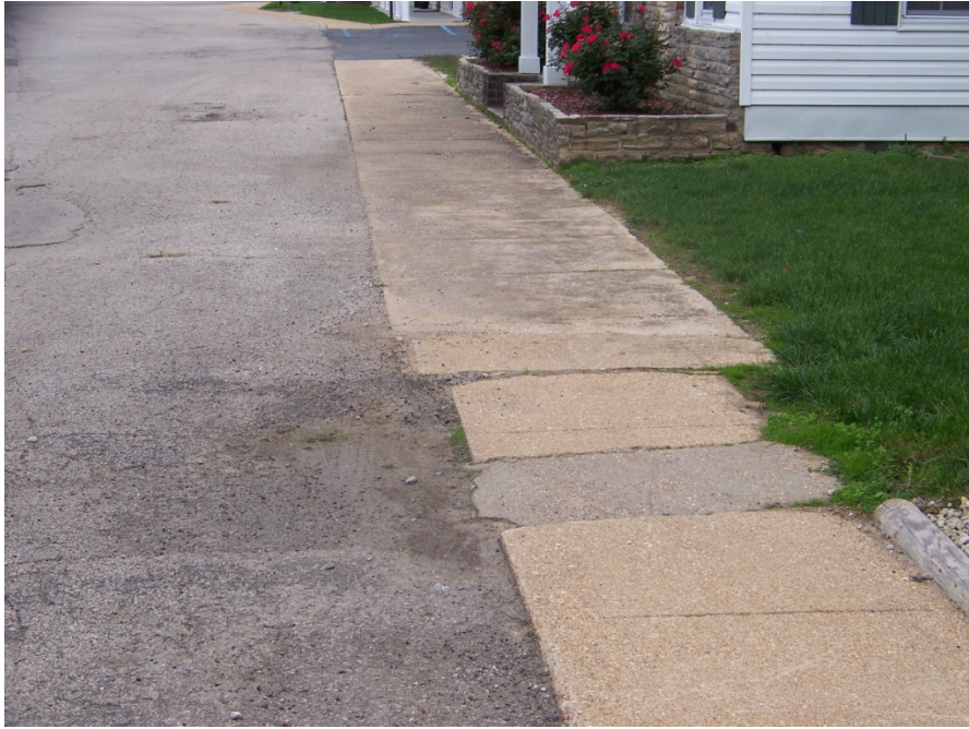
Fair Condition: Cedar Street, south side looking east from Hickory Street
