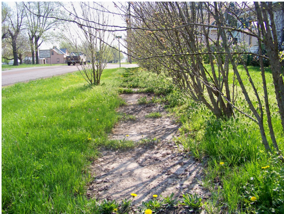
Poor Condition: First Street, south side looking east
