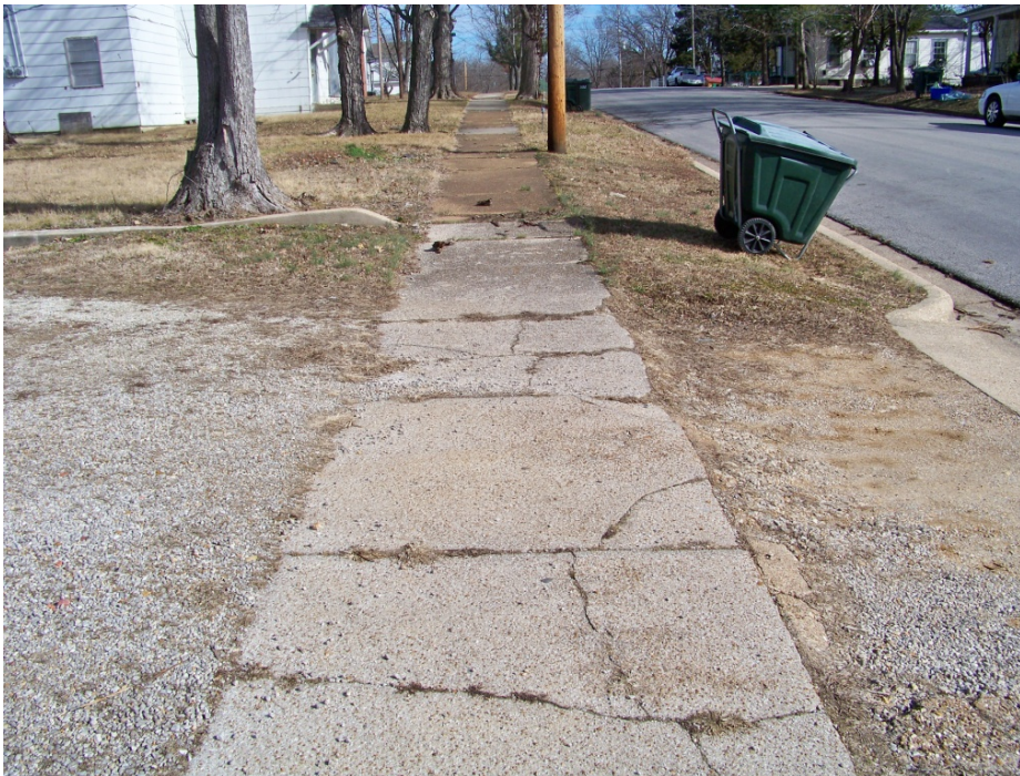
Sidewalks on portions of Olive Street are in poor condition.
