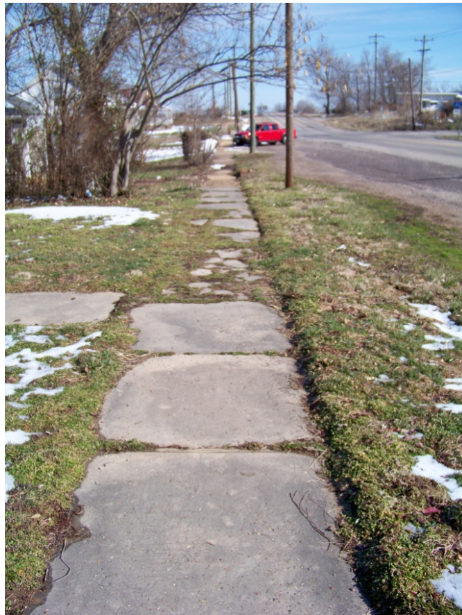
Poor Condition: E. Pine Street, west side looking north toward N. Old U.S. Highway 66
