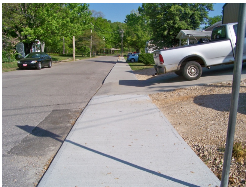
Good Condition: Olive Street, east side looking north
