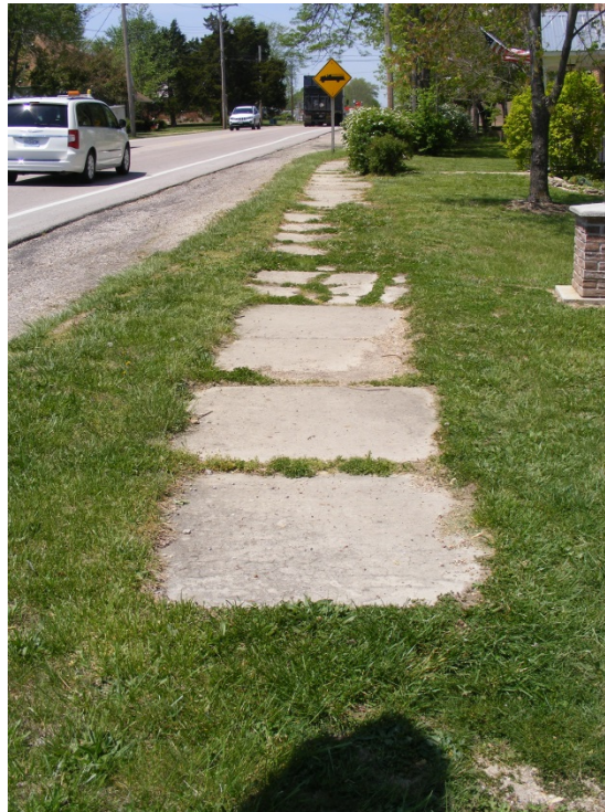
Poor Condition: Intersection of Highway 50 and 1 st Street, northwest corner looking east.
