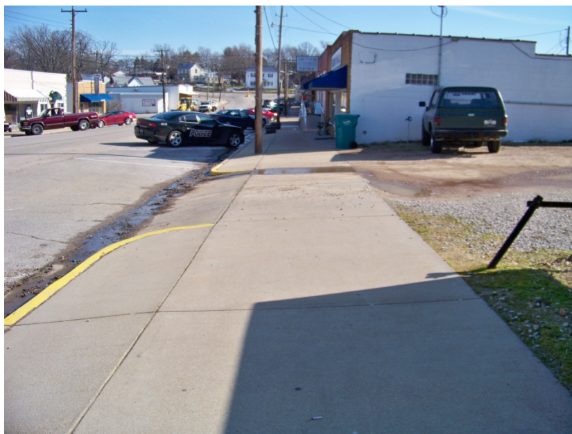
Good Condition: E. Pine Street, south side looking east toward Walnut Street
