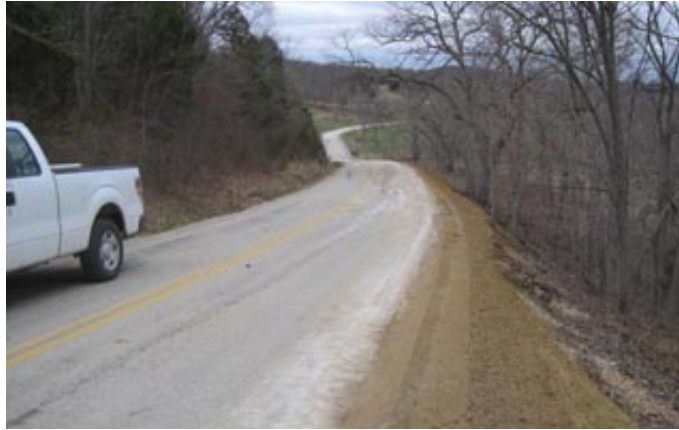
Route N after improvements by MoDOT
